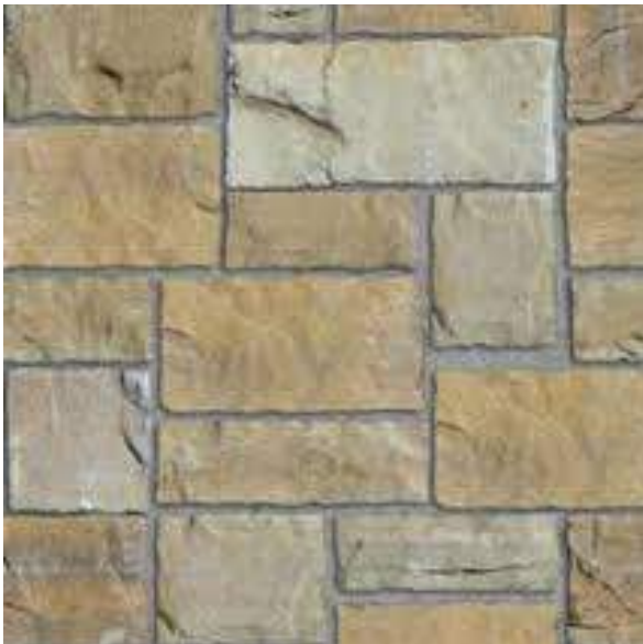
(2): ANCHORED CAST STONE MASONRY
